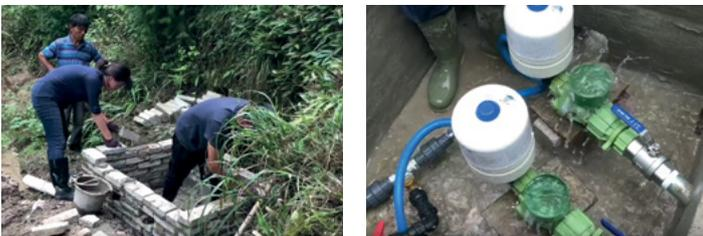
The system was installed and will be maintained by the local community. The villagers built a supply tank and pump chamber with rendered block work. They also laid the steel Supply Pipes and mdpe delivery pipes up to the village.
